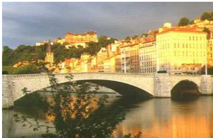
Bridge over the Rhone river
